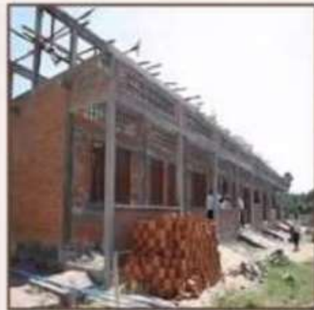
School Bldg. Construction
